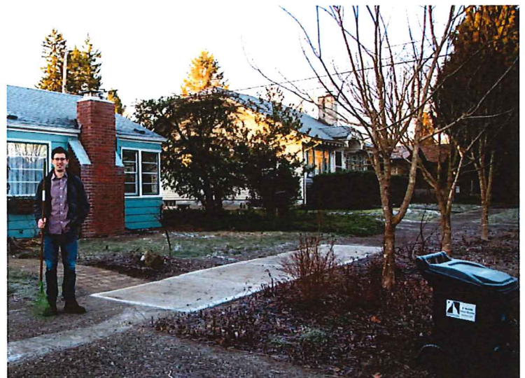
Sidewalk replacement work completed by a contractor, hired by homeowner.
