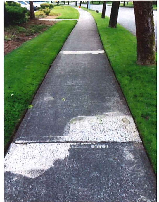
A sidewalk that's been repaired by grinding.
